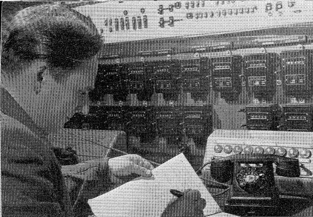
At the control panel of a transfer line in an automated factory, where the machines do the hard work.
