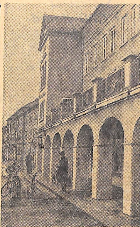
The Government of the German Democratic Republic shows the greatest concern for the working people. Housing construction on an extensive scale is being carried out in the Republic. Above are some new houses for miners in the town of Lauchhammer.
