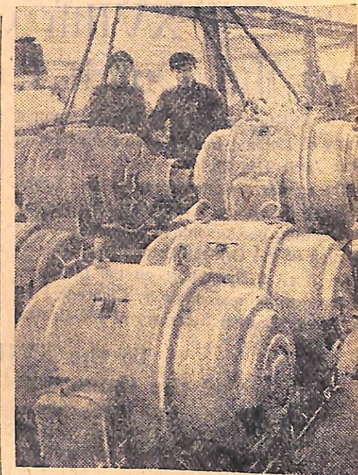
This year the first stage in the construction of China's biggest state plant of electrical equipment in Harbin will be completed. A number of shops have already been put into operation. Above: Finished products of the plant.
